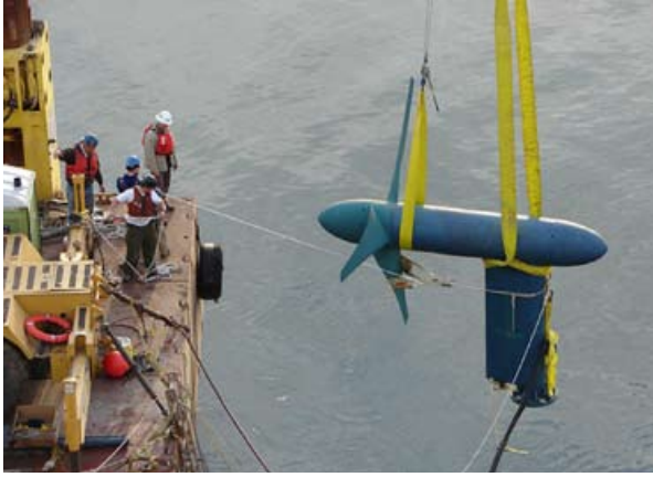
Engineers installing a kinetic hydropower turbine underwater with no dam
